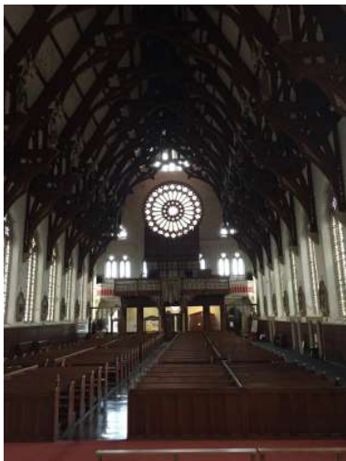
Left: St. Walburge Church Interior's 'Hammer-beams'
